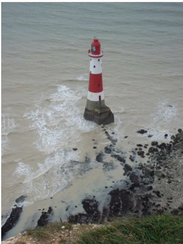
Beachy Head Lighthouse, Eastbourne, England N 50° 44.026 E 000° 14.488
